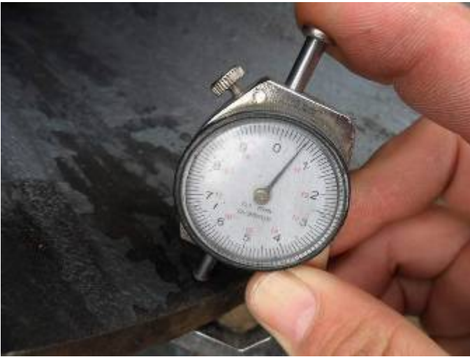
21. Wall thickness test : 10.8mm
