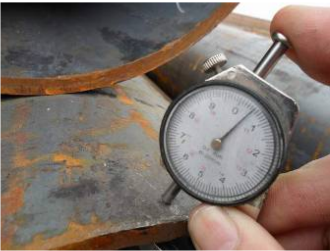
27. Wall thickness test :10 .6mm
