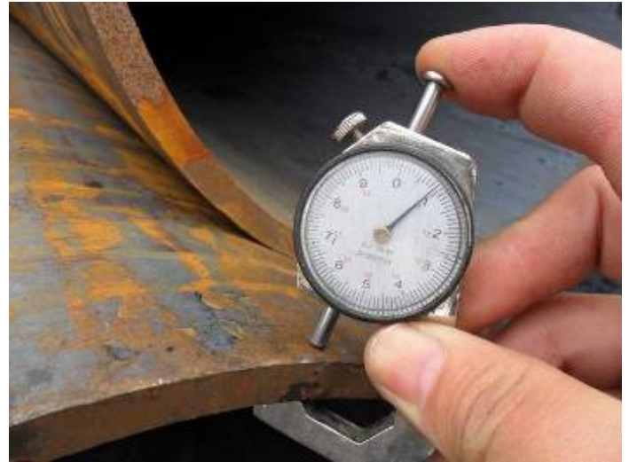
22. Wall thickness test : 10.9mm
