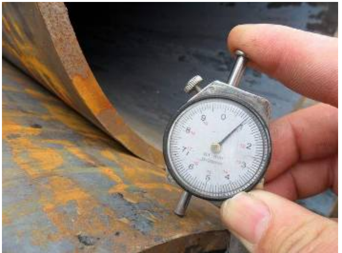
24. Wall thickness test : 10.8mm
