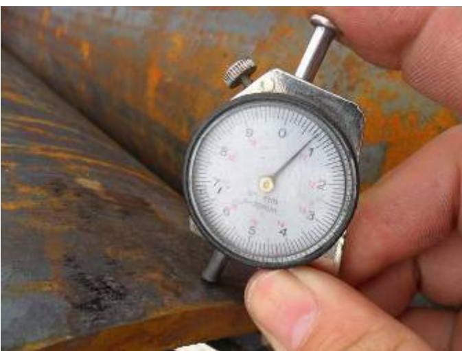
25. Wall thickness test : 10.4mm
